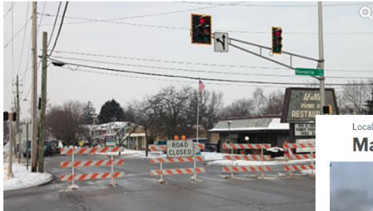
A water main broke along State Boulevard near Parkview Hospital on Friday, Jan. 5, 2018.
