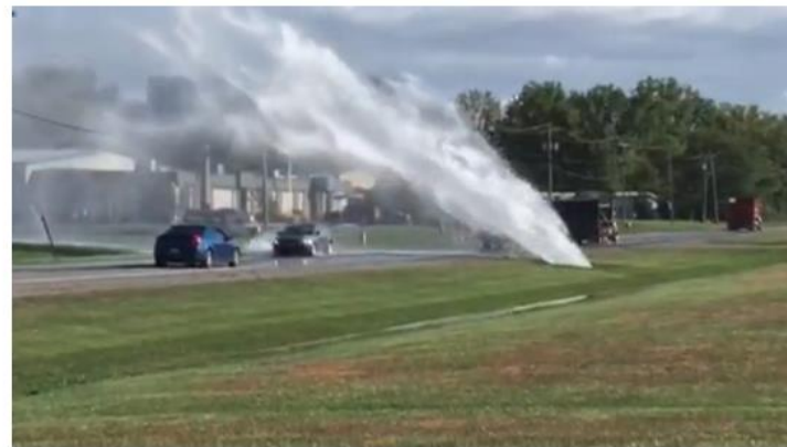
FORT WAYNE, Ind. (WANE) A water main burst in southern Fort Wayne and a geyser is shooting water high into the air.
