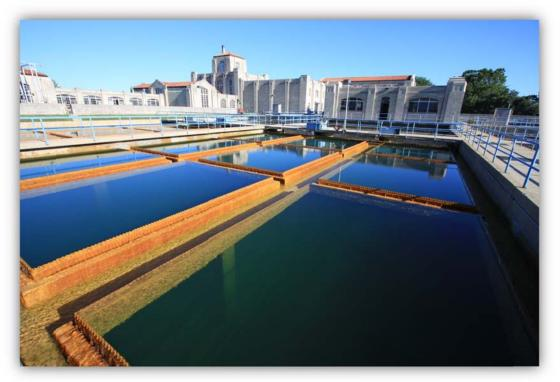
The floc clumps continue to grow and pick up the carbon and other suspended particles. Water flows into settling tanks where the clumps of floc are so heavy they settle to the bottom and clear water flows out from the top. This process of flocculation and settling happens two times.
