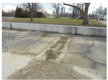
Photo 11 – Filled pit in southwest corner of the southwest building foundation on the site
