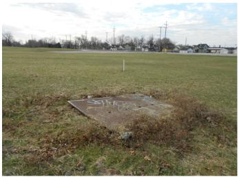
Photo 13 – Typical steel plate over storm water drains across the site; Note groundwater monitoring well in background
