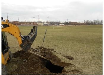
Photo 15 – Uncovering southeast steel plate located beneath cover of fill material on the site
