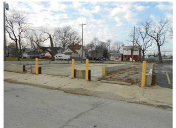
Photo 10 – View of building foundation on the southwest corner of the site looking to the southwest; Note filled truck dock in near corner
