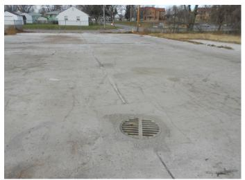
Photo 7 - Floor drain/sump in northwest building foundation
