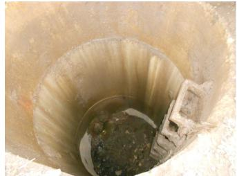
Photo 16 – View of storm drain manhole beneath the southeast steel plate
